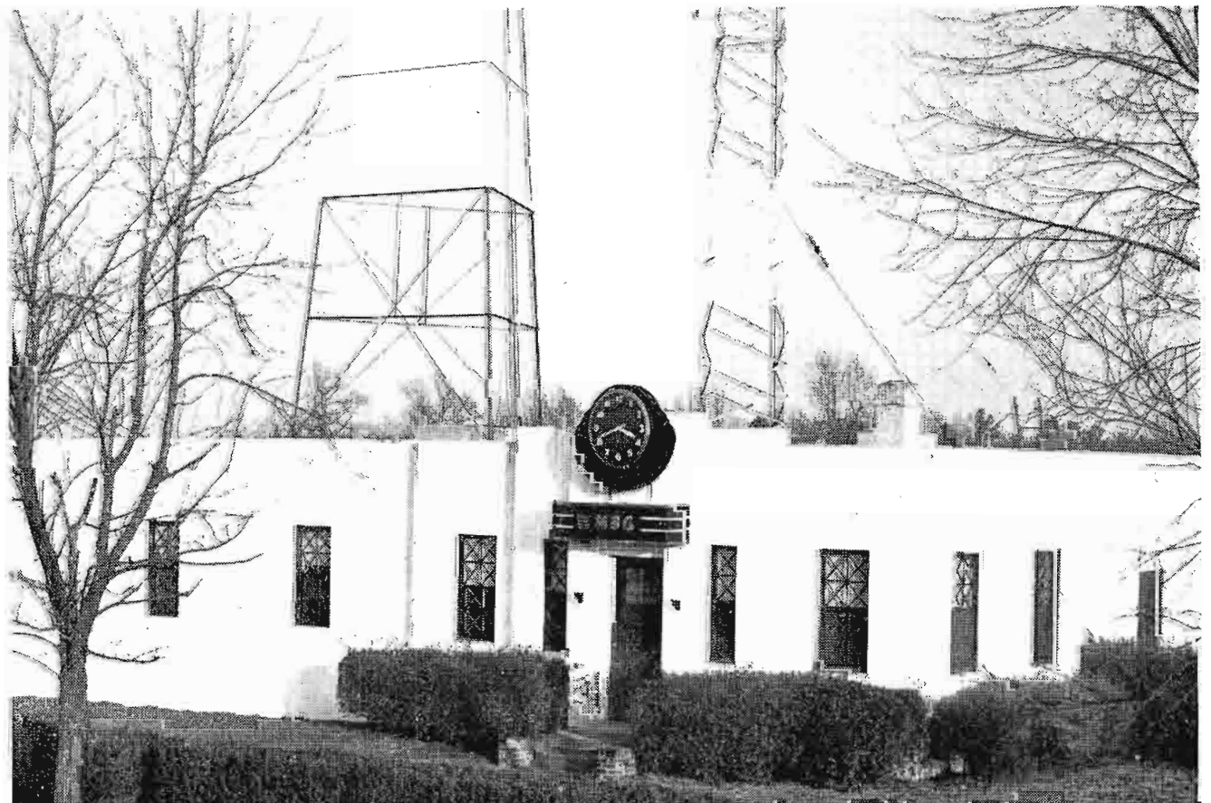
Picture (at left) is view of WTVR 642-foot auxiliary tower and RCA Superturnstile Antenna. The WTVR auxiliary transmitter building below houses complete auxiliary audio and video facilities. These facilities can be placed into operation instantly upon a failure at the main transmitter location. Signal is micro-waved from studio to auxiliary transmitter by RCA Link.
