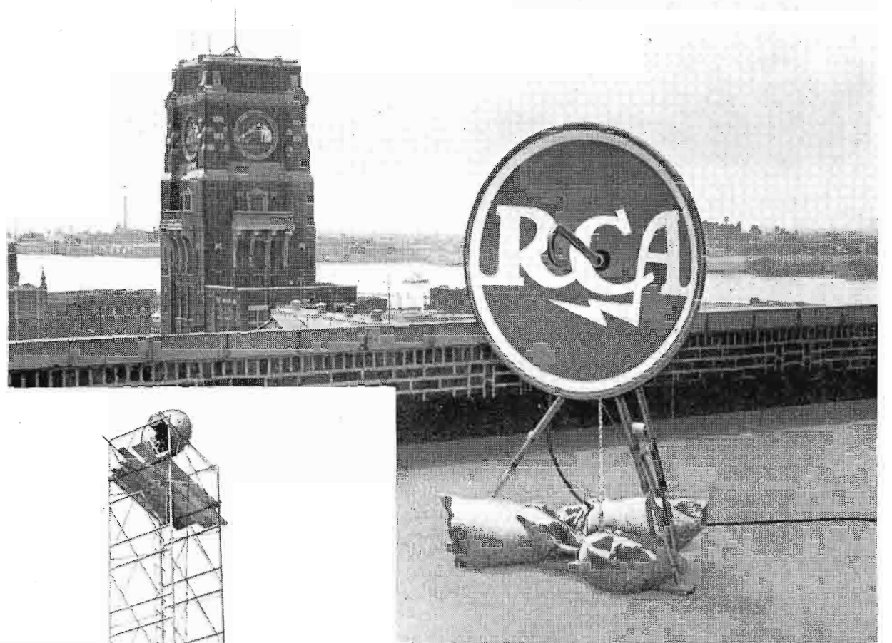
FIG. 6. Microwave installation used for closed-circuit TV tour of Moorestown Plant staged for nation's ranking air chiefs. Above, 4-foot parabolic antenna is moored to roof of RCA's general office building in Camden; below, temporary 70-foot tower on Moorestown Plant from which signals were relayed.
