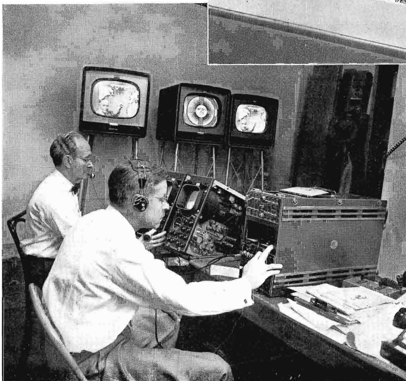
FIG. 3. Two camera-chains in AT&T stock-owners room relayed proceedings to overflow audiences in five nearby rooms at 196 Broadway and also cut into televised program at Long Lines building during final sequence. The cameras are shown on right. Note TV receivers lining room, and RCA PT-100 large screen theatre TV equipment on far balcony which brought TV show to stockholders. Theatre TV projectors on both balconies projected program on two large screen (seen above cameraman) which were lowered at time of show.
