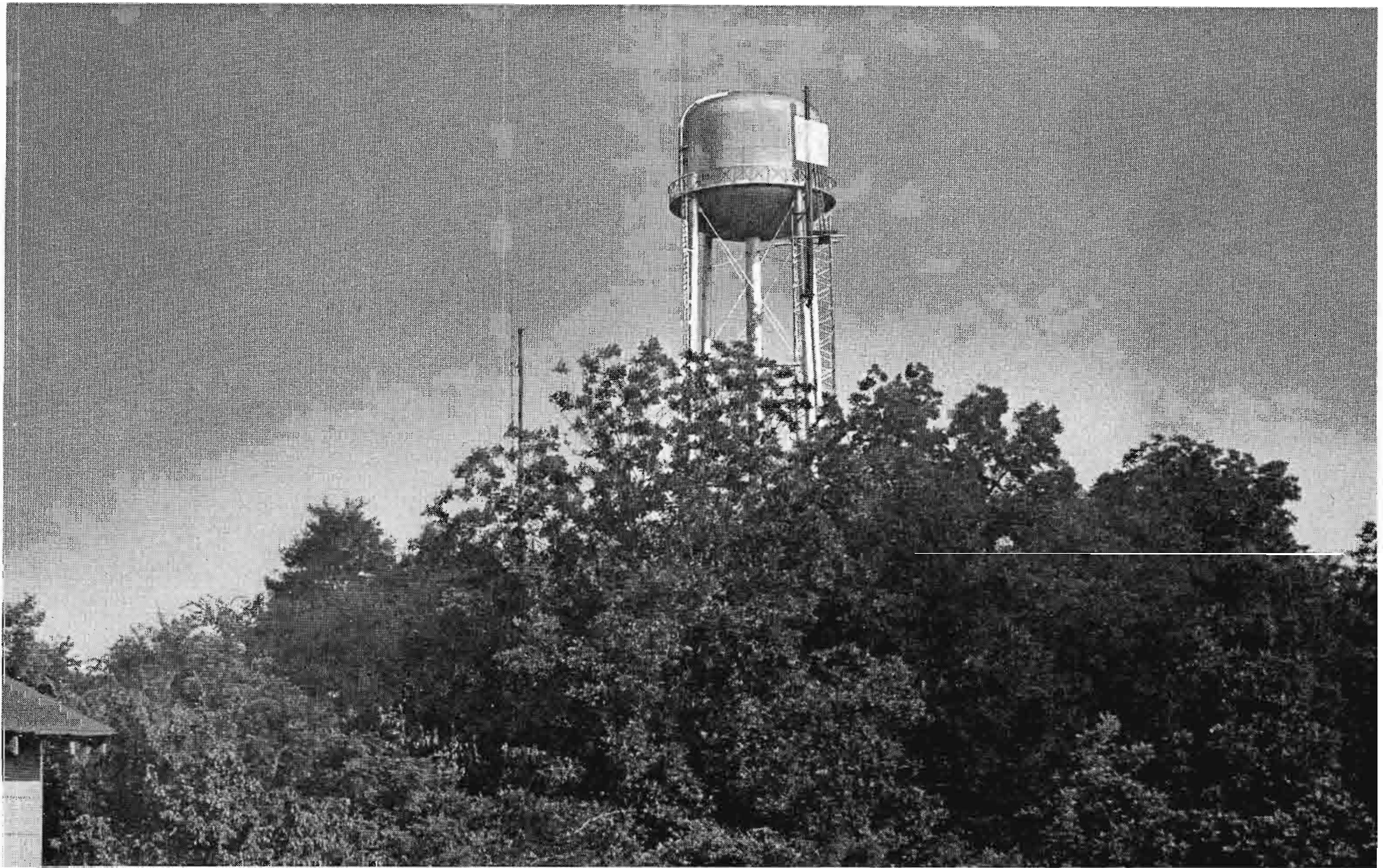
FIG. 6. The KK2XFI Booster was installed on a slight elevation about two miles northeast of the center of Vicksburg. The view above shows the square zig-zag receiving antenna mounted on a 110-foot water tower, and the vertical zig-zag transmitting antenna mounted on a 90-foot pole to the left. The two antennas are about 100 feet apart.
